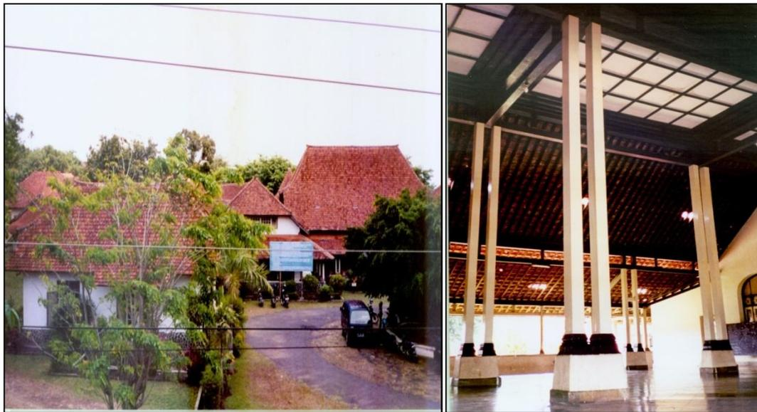
Figure 6: School van Deventer now SMU Semarang Kartini and interior multipurpose building. Thomas Karsten designed the building in 1923. In the multipurpose building houses a development Limasan Lawakan home form with saka guru (main columns) shaped double column. (Source: Ardiyanto documentation, 2005)
