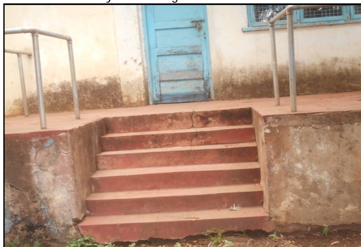
Figure 2: Steep stairs in SC3 in the students' library
